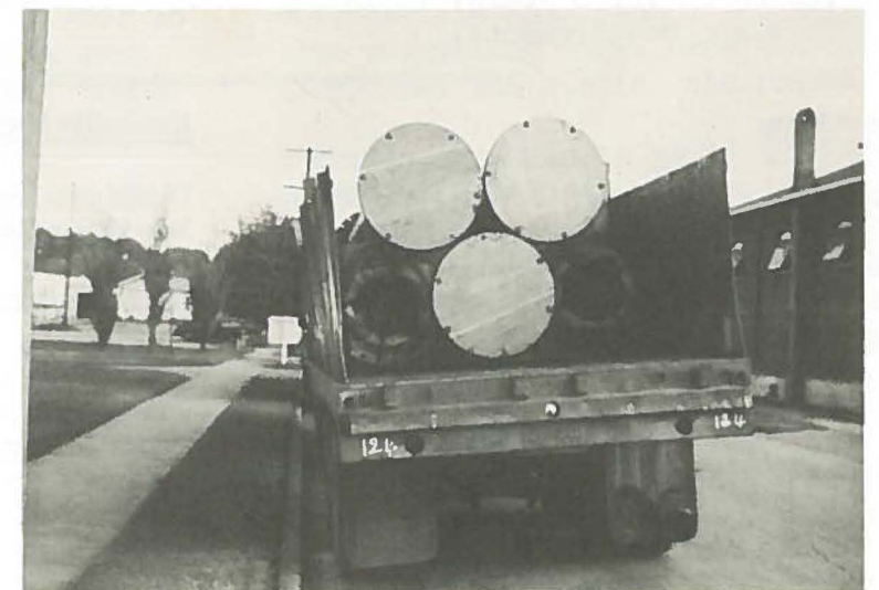
At right: A truck loaded with River-Crossing pipe leaves the National plant - each length of pipe weighed approximately 5500 pounds.
