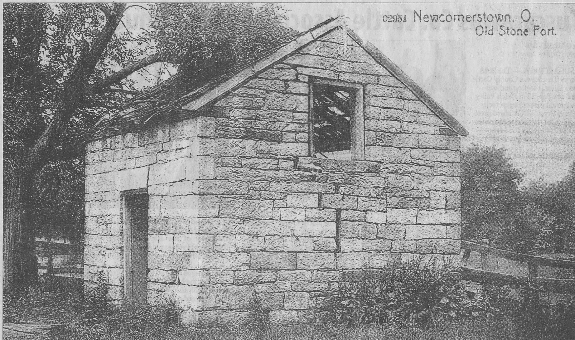
The old Stone Fort seen in this 1900s postcard view, was once part of the town of Evansburg. The fort was the only remaining structure after a cyclone wiped-out what was left of the town in the late 1890s.
