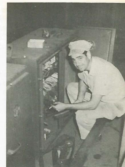
Electrician, EDWARD BROWN, works on the Melting Dept. crane controls.
