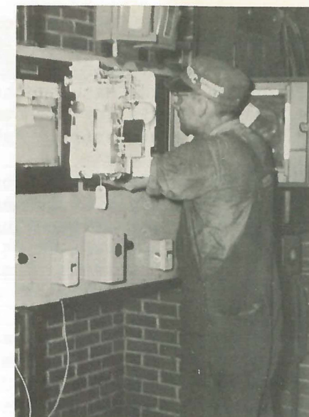
EUEL JACKS installs new annealing oven controls in the deLavaud Foundry.
