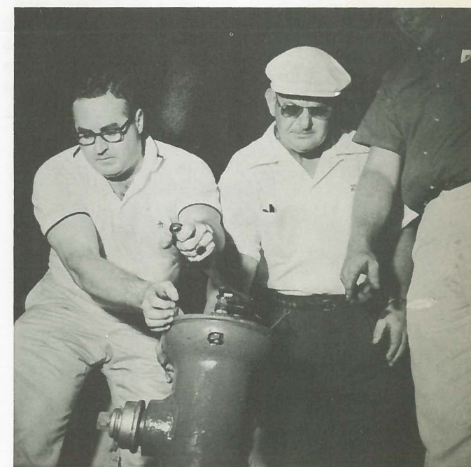
BOB HOLZ of Minneapolis, left, and HOWARD BECK of Dallas, very carefully adjust the drain mechanism before a final test to determine the accuracy of their job.
