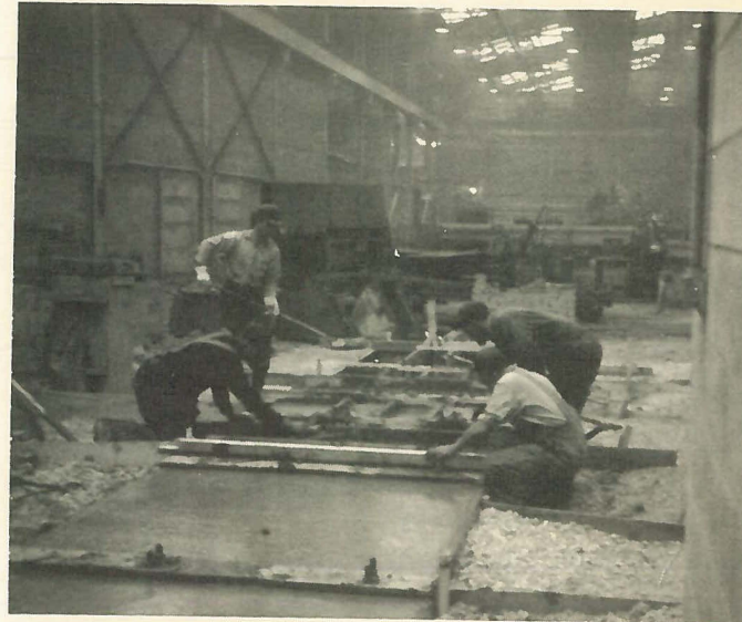
POURING FOUNDATION FOR MOLD GRINDER INSTALLATION
