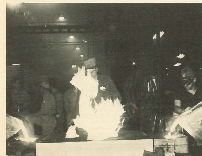
Assistant Foreman KENNETH GUTHRIE watches closely the pouring of SHERMAN'S first 36-inch case. The flame in the center of the photo is caused by burning gases which escape from the mold.
