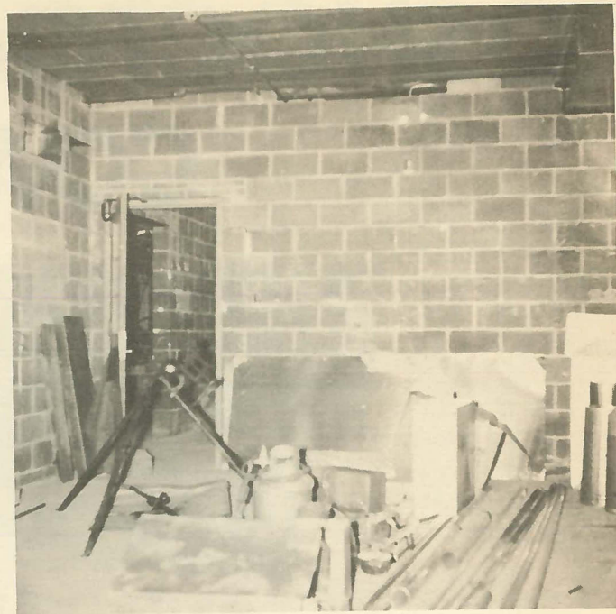
Inside work progresses on the Laboratory addition at Coshocton.
