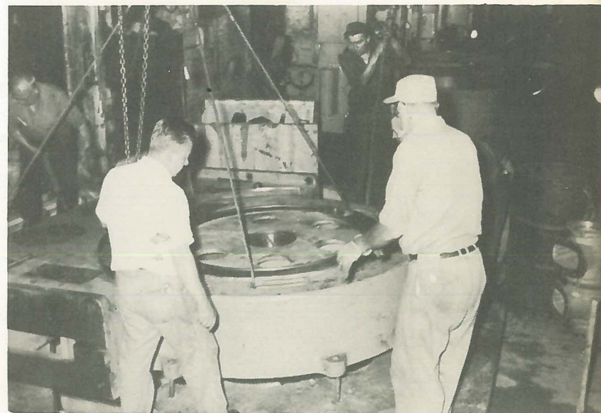
Pictured left, Joe Sliwinski supervises the lowering of the base over the anchor bolts as Armond Plouffe operates the hoist in the background.....
