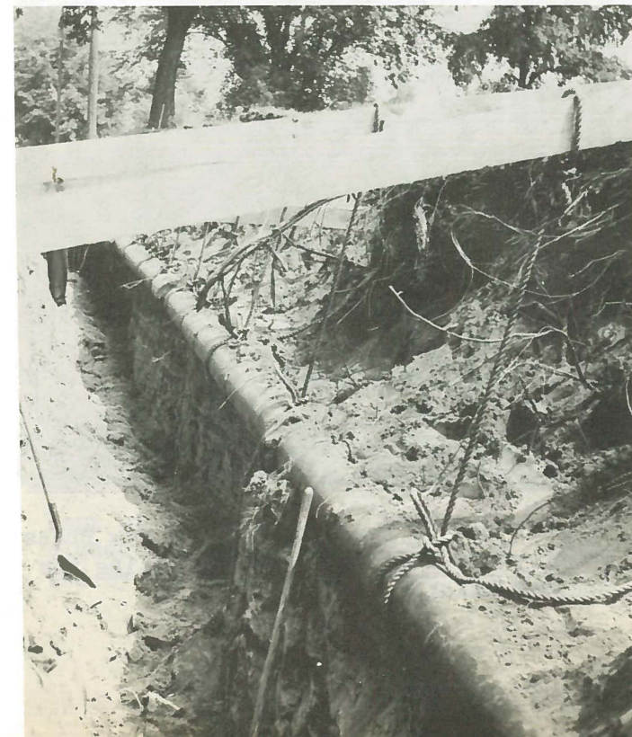
Below, shows pipe, ready for lowering into trench at new grade.
