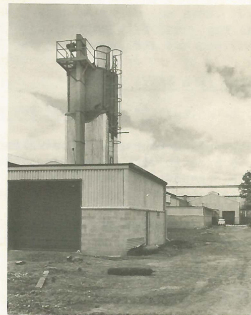
Bulk cement and sand storage area.
