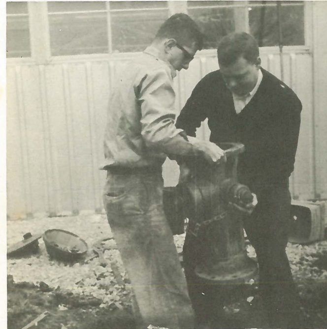
Salesmen Ed Powers and Ed McMahon were busily engaged in extending one of the fire hydrants located alongside our plant. This is a part of the sales training extended to sales trainees at the factory.
