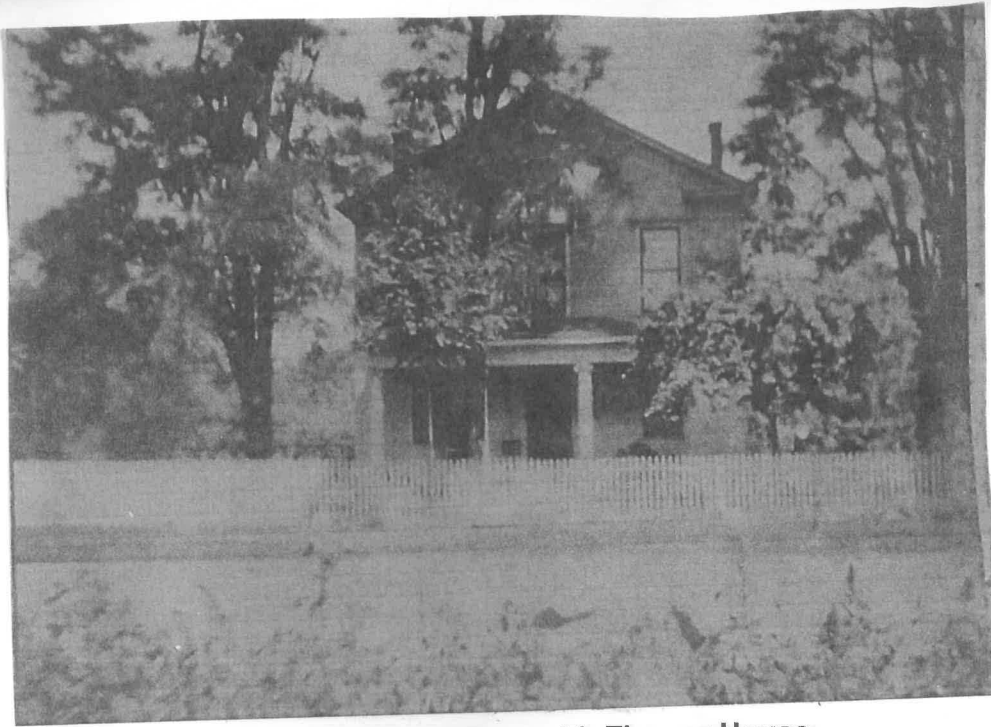
E. State St. East of Route 21 Zimmer House
