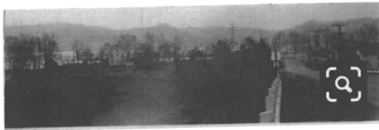
Viaduct looking south - flood 1937 - Newcomerstown, OH
