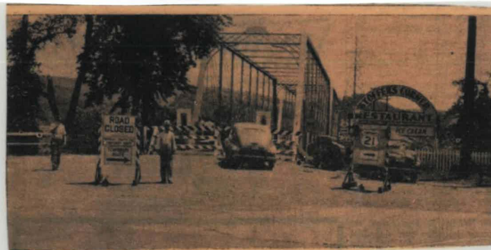
Aug 5, 1948 Bright Studio: PILLING ST. BRIDGE , closed for repairs last week, has necessitated a detour for Route 21 traffic as well as for residents of the area south of town. When completed early in September the bridge will be safe for at least 15 tons. Local residents hope eventually for a new, wider span across the Tuscarawas river.
