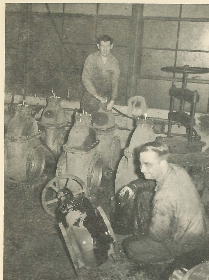
HAROLD BORNT pauses in his brush swinging duties while STAN ZUMBACK, in the background, bolts a follower into place on a 12" valve.
