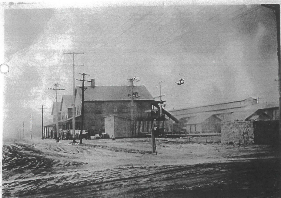
TEMPORARY CLOW SUBSTATION NEWCOMERSTOWN FEB. 23, 1924
