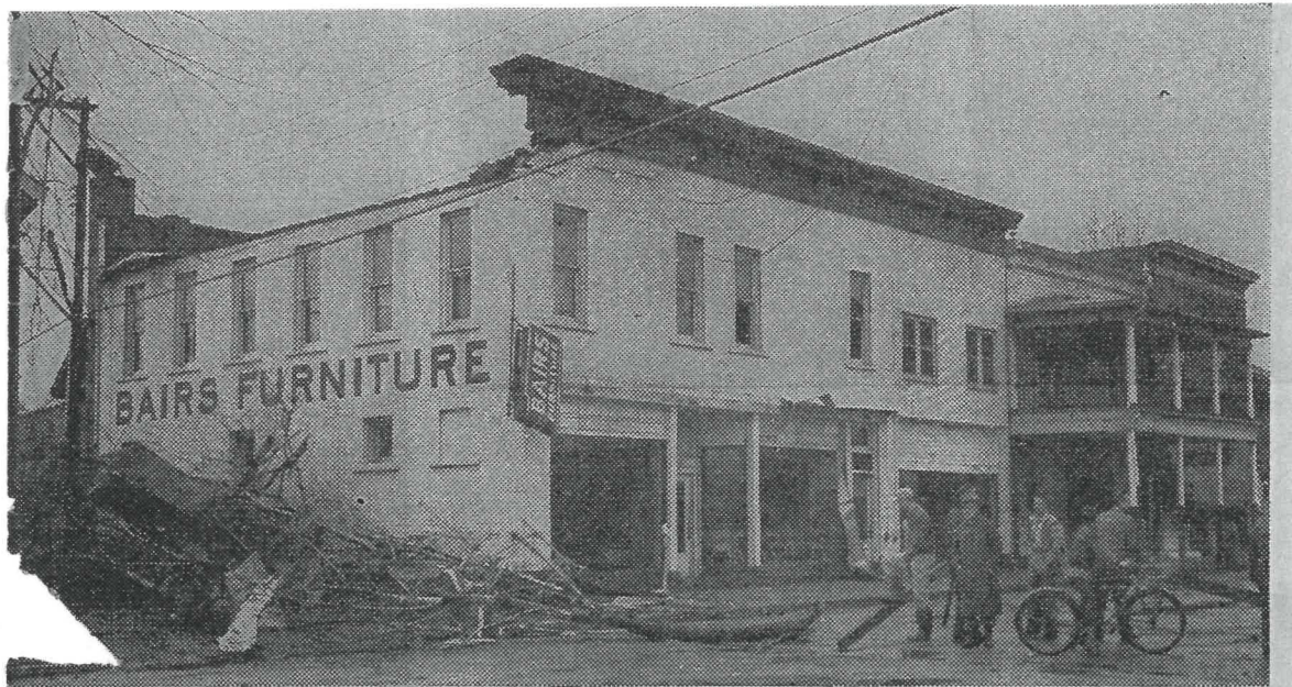
BAIRS FURNITURE BUILDING was heavily damaged in the Friday storm as winds knocked over the fire wall and ripped off the roof. An upstairs apartment was virtually wrecked. Plate glass windows were knocked out.
