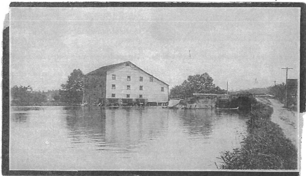
Mill on the Canal
