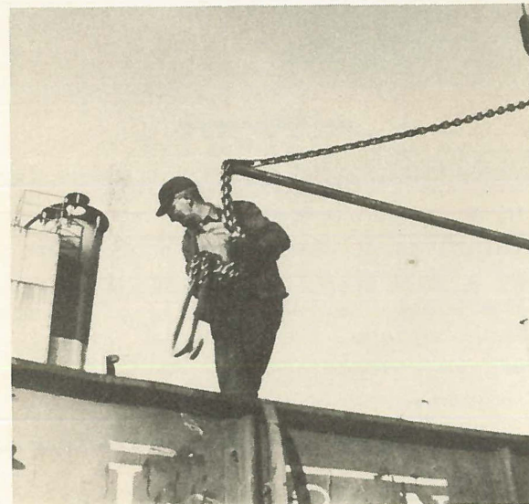
Dave Van Haaften is ready to hook another length of pipe for unloading.
