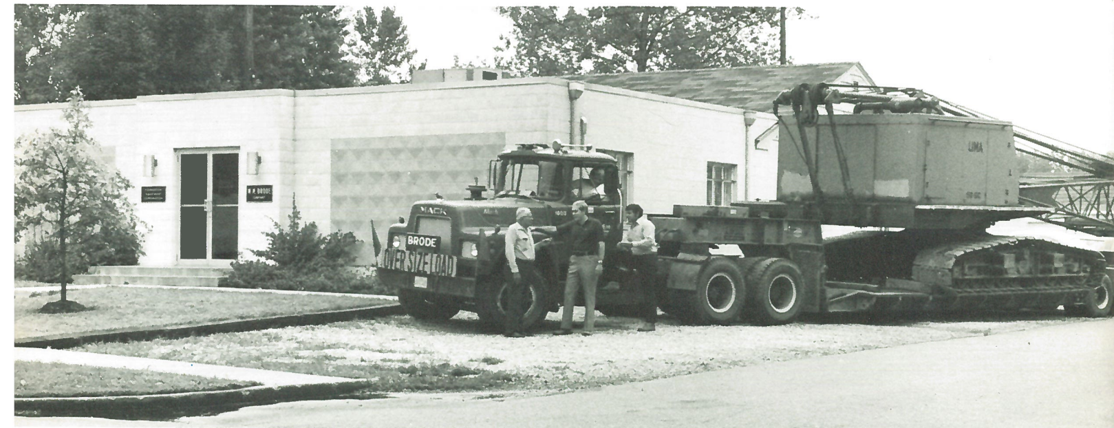
Erwin Johns, retired general superintendent (left), George Brode (center), and Robert Brode (right) pose in front of the company's modern offices completed in 1972.
