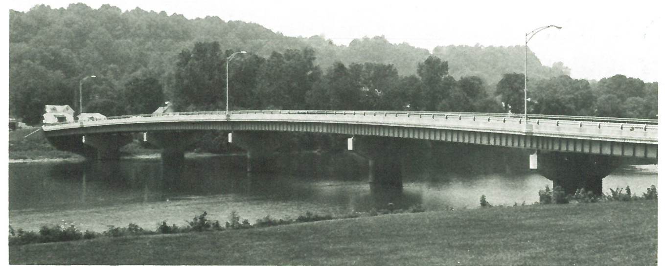
1968 — HIGHWAY BRIDGE — carries State Route 78 across the Muskingum River at McConnellsville, Ohio. Job for Ohio Department of Highways.
