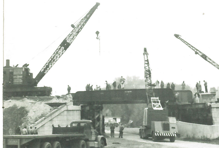
In 1955 Whipple, Ohio: another Pennsylvania R.R. underpass.
